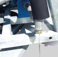
Self-draining spray manifold and discharge pump plumbing
