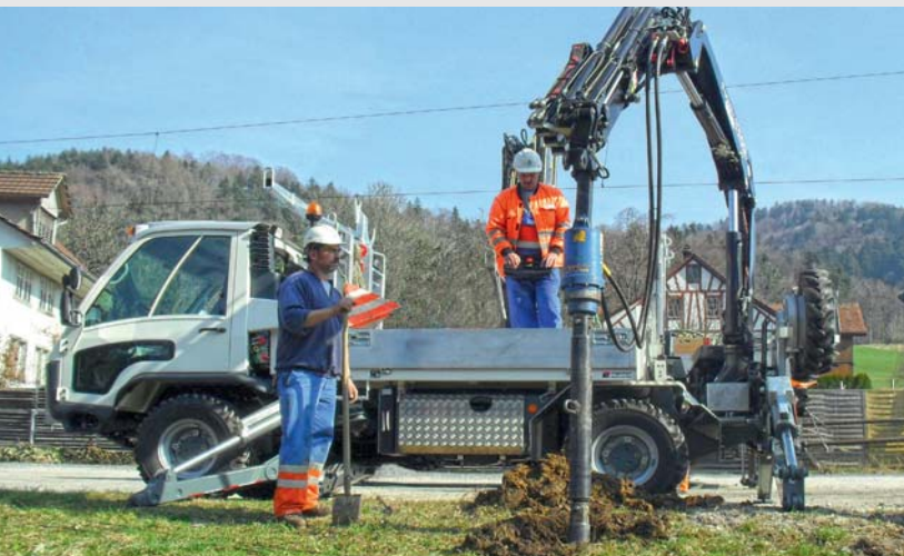
Aebi VT450 Vario crane with earth drill
